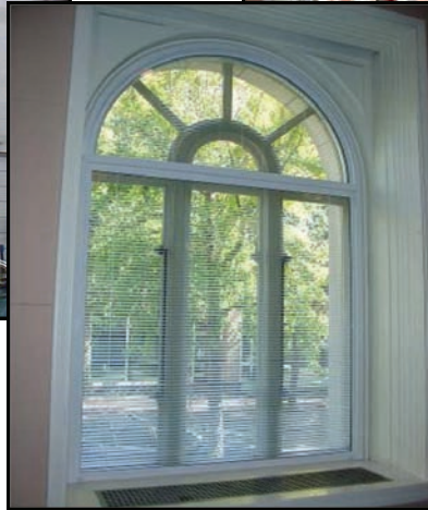
Interior Retrofit Blast Window
